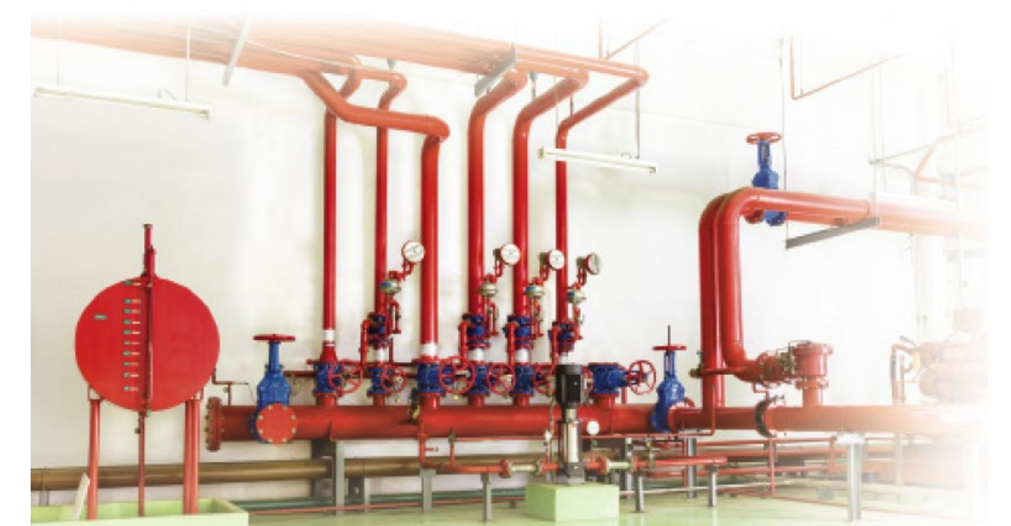
Figure 37: Fire water supply systems.
