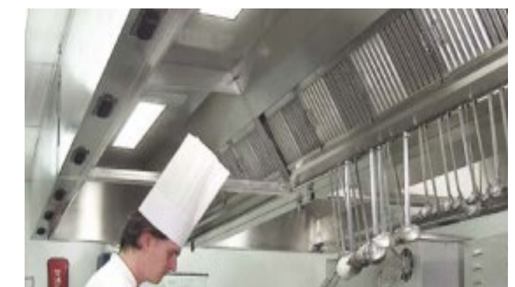
Figure 9: Exhaust flows from cooking hoods can be variable based on cooking activity with local non-treated air supply (compensated air hood).
