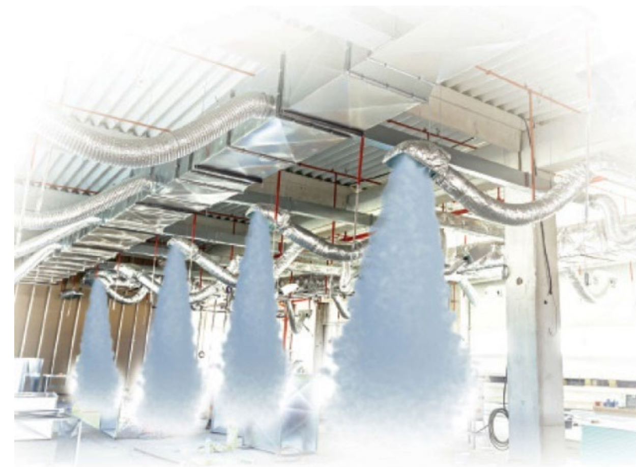
Figure 43: Foam system.
