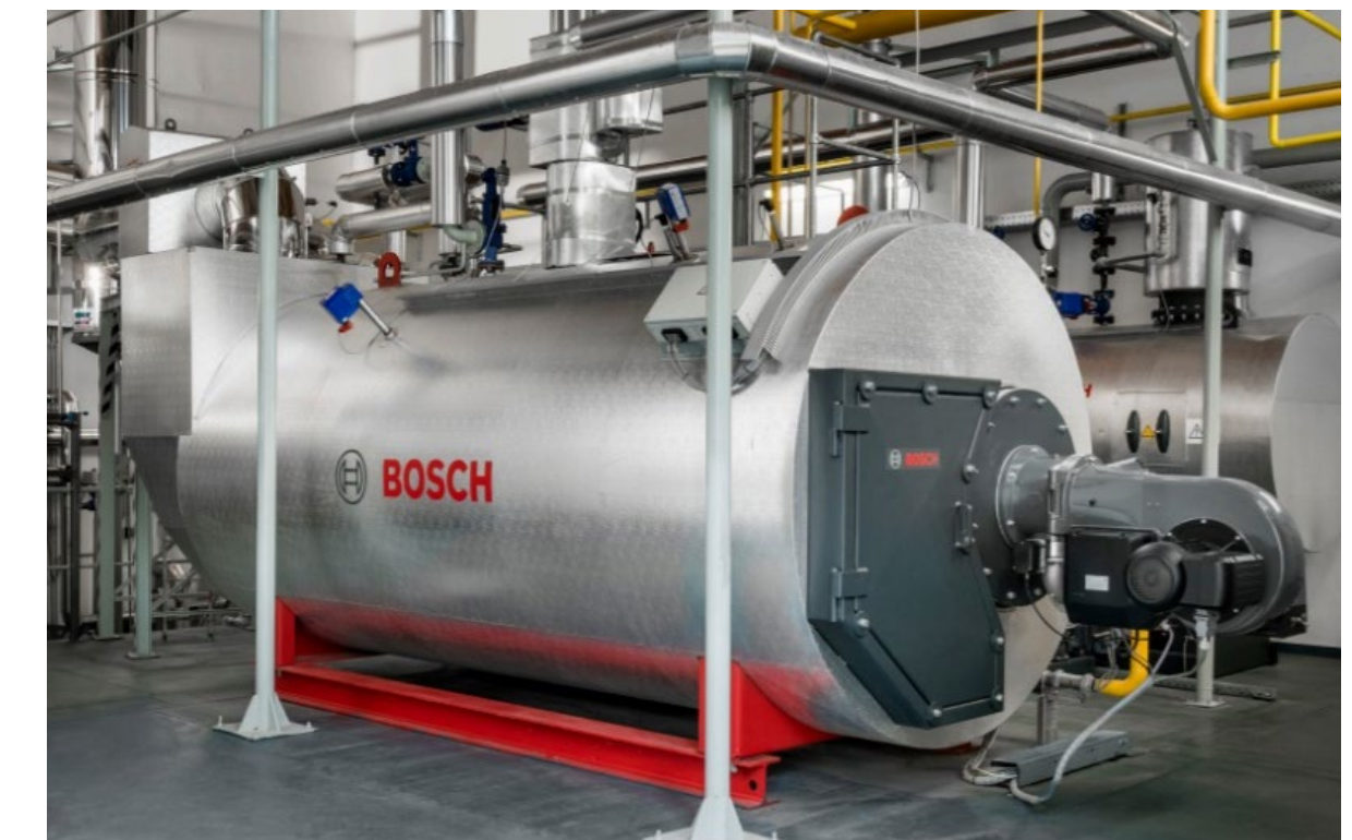
Figure 19: Steam boiler. Source: Bosch thermotechnology™.
