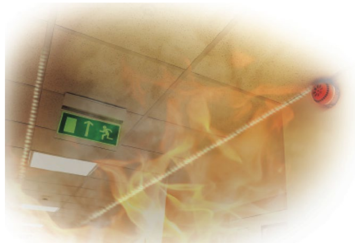
Figure 47: Emergency lighting system.
