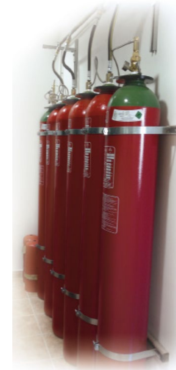
Figure 44: Fixed Powder Extinguishing system.
