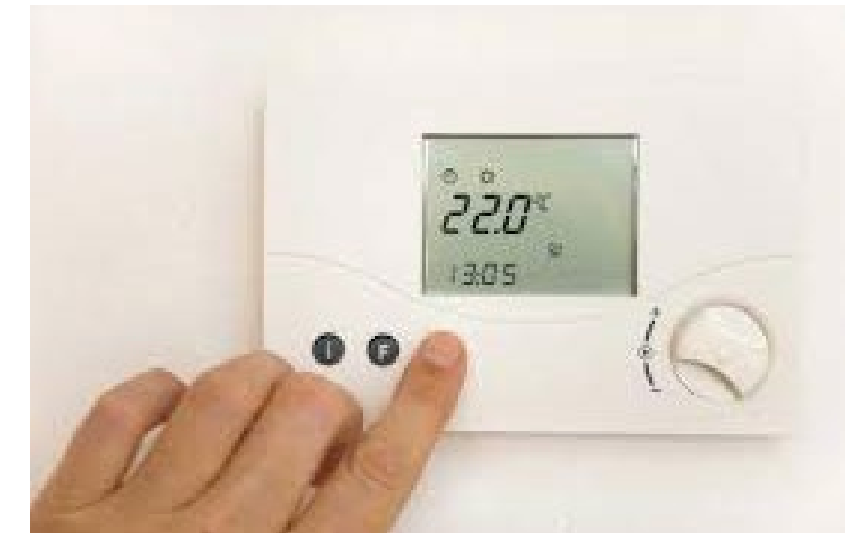
Figure 18: Review of room temperature configurations can help with energy efficiency. For example, in non-healthcare areas, the room temperature set point can be set to 26 °C in summer and 20 °C in the winter.
